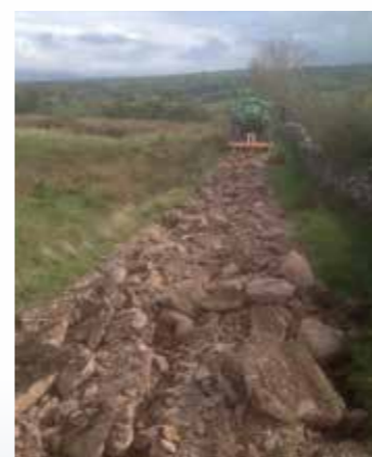
The road having been ripped up before crushing
